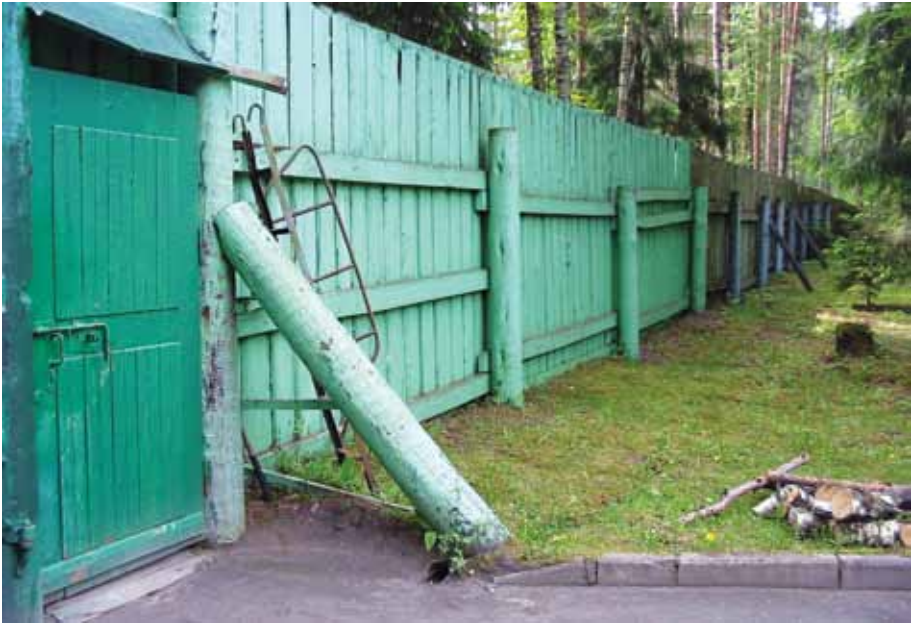
Gate and fence (interior view). 2008
